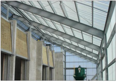
Fertilizer storage facility installed with Enduro DuroLite roofing & siding panels
